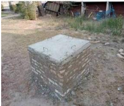
Fig.1 a- RCC roof
