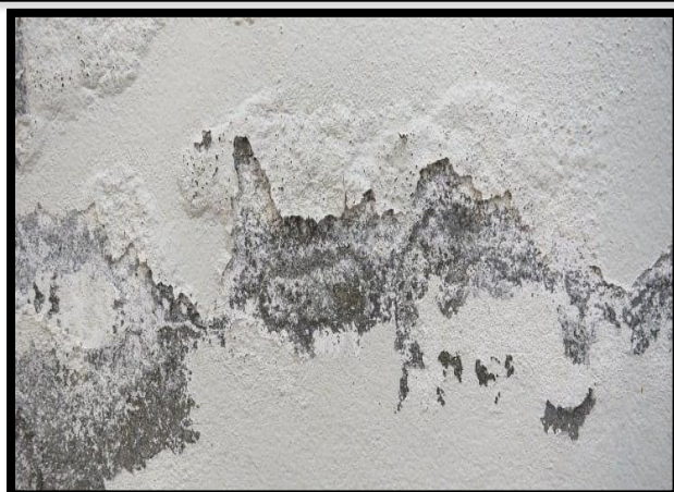
Fig.5: Evidence of Water Seepage in Coastal Apartments Karachi, Pakistan
