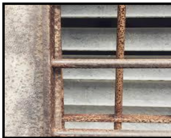
Fig.7: Evidence of Rust on Grills in Coastal Apartments Karachi, Pakistan
