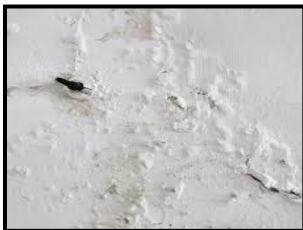
Fig.6: Evidence of Water Seepage in Coastal Apartments Karachi, Pakistan
