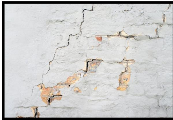
Fig.3: Evidence of Plaster Cracks in Coastal Apartments Karachi, Pakistan
